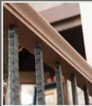
Iron Balusters Installed to handrail
