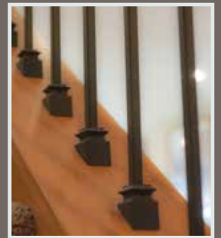
Iron Balusters Installed with pitch shoes
