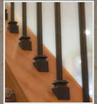
Iron Balusters Installed with pitch shoes
