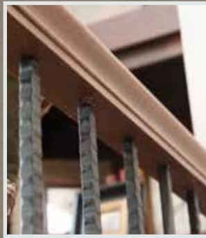
Iron Balusters Installed to handrail
