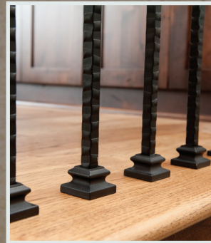
Iron Balusters Installed to hardwood floors with flat shoes
