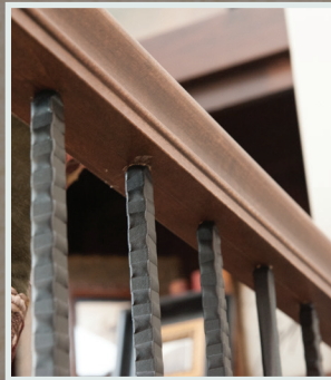
Iron Balusters Installed to handrail
