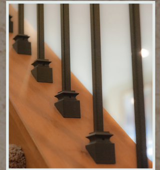
Iron Balusters Installed with pitch shoes
